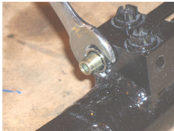
Fig 6-4 Valve with cap removed
