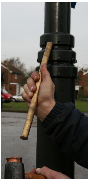
Fig 5-25 Removing cap
