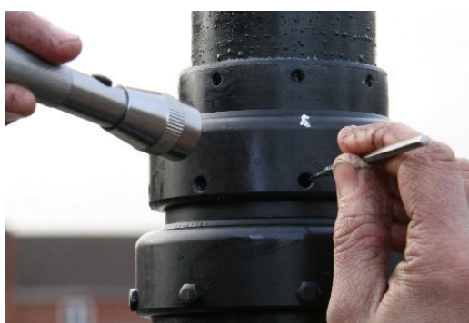
Fig 5-29 Checking for debris
